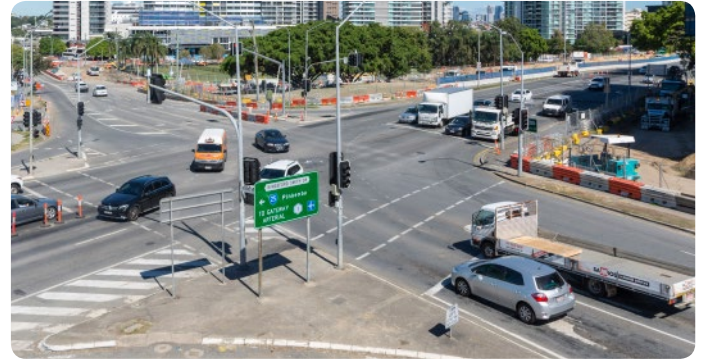
Nudgee Road intersection - April 2017
