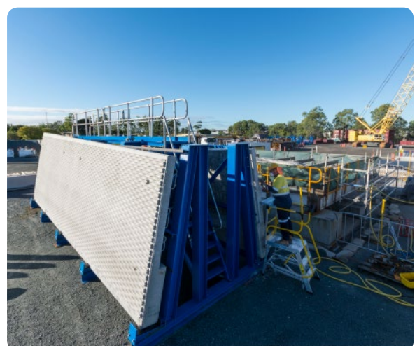
Production of fascia panels at Morningside - April 2017
