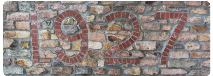
1927 insignia in the retaining wall adjacent to Remora Road - June 2017
